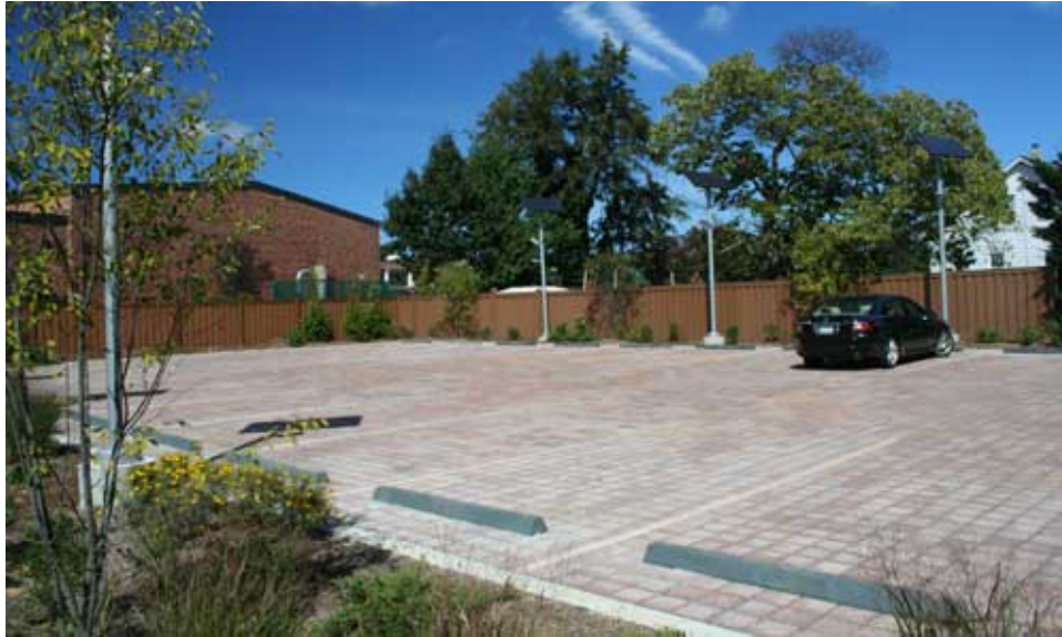
Photograph. Alternative stormwater management techniques such as permeable pavement and vegetated swales, like those constructed at the Lindenhurst Memorial Public Library shown above, could significantly improve ground and surface water quality.
